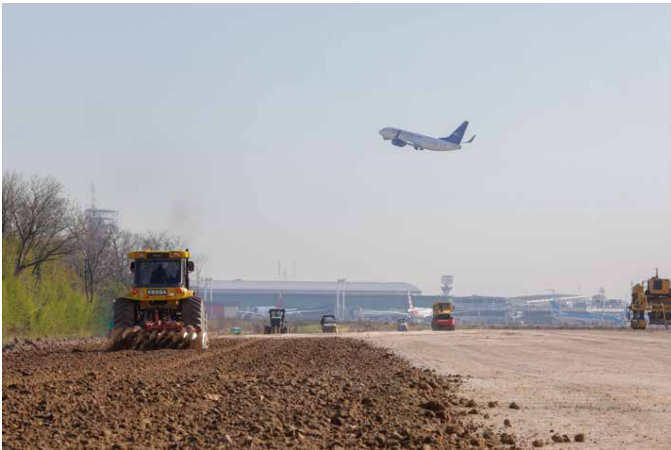
Work of prologue of the taxiway to header 35 in airport Ezeiza
