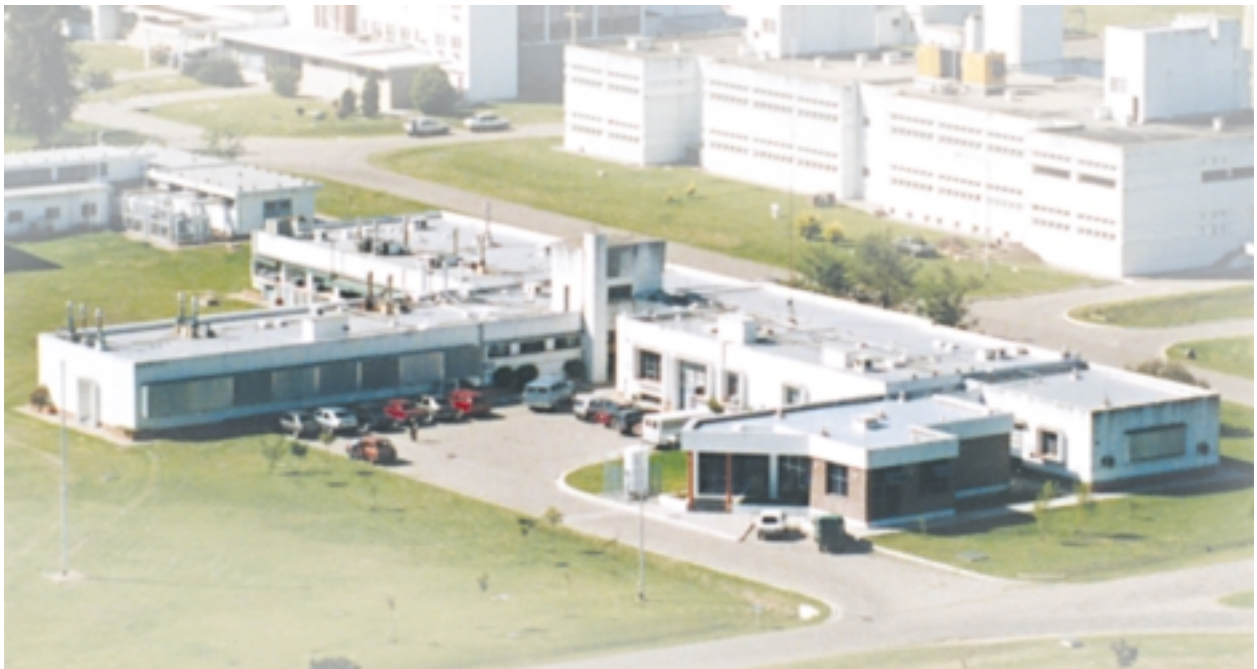
The ARN building at the Ezeiza Atomic Center
