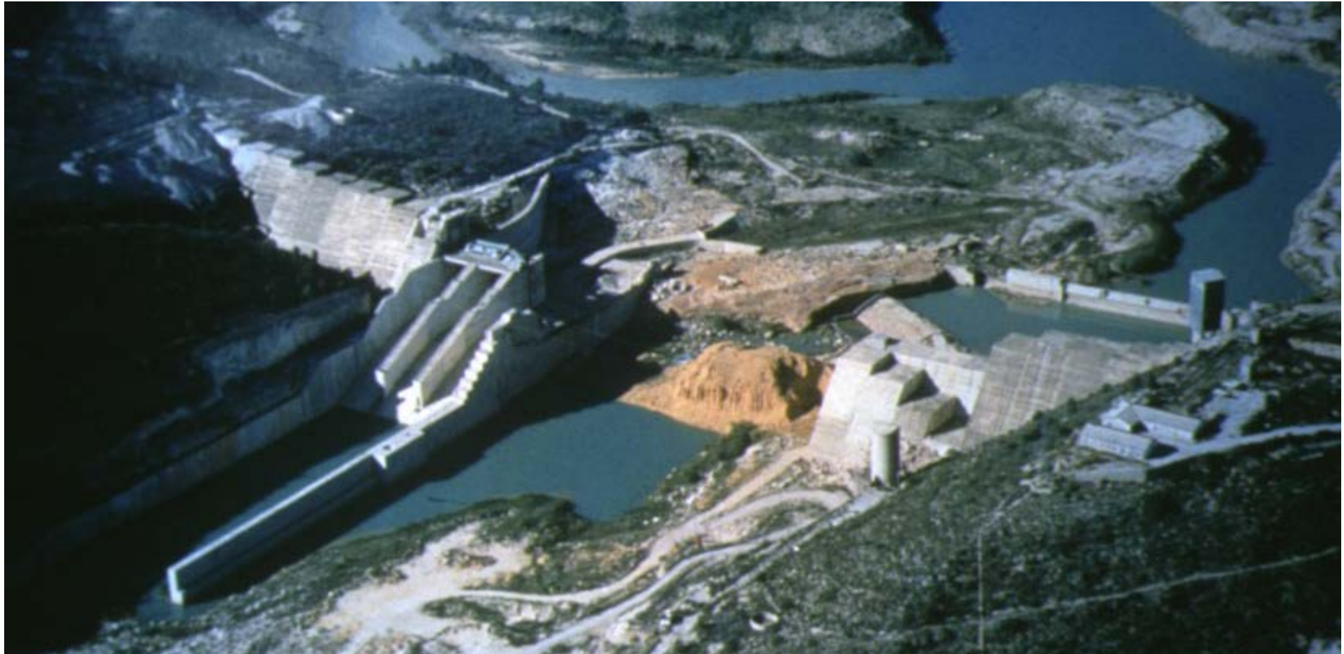
Picture: Failure of Tous Dam, Valencia, Spain, 1982
